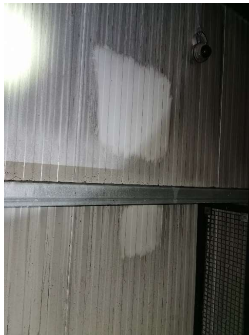
24. Cleaning test panels in Unit 2a.
